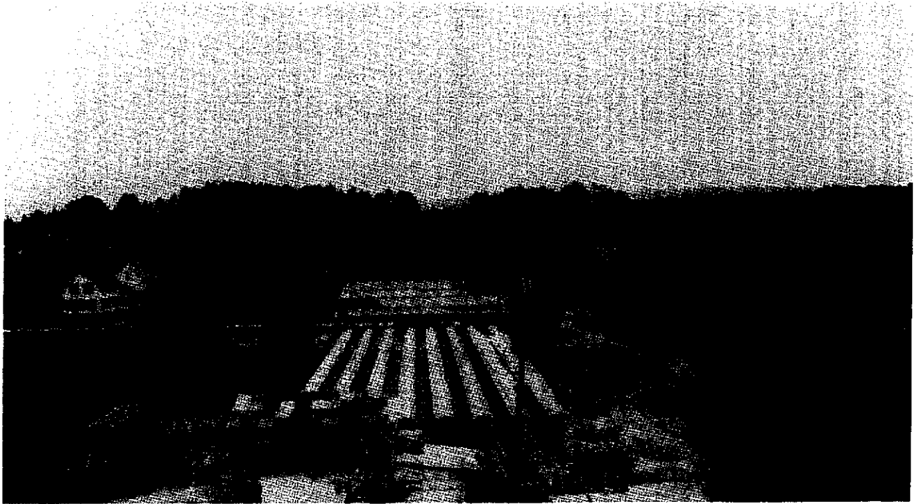
Figure 11. Samuel Holt brickyard, Concord, New Hampshire, c1925. By the early 20th century, a number of New Hampshire brickyards had steam- or electric-powered pug mills and soft mud machines, here housed under the sheds in the foreground. Such yards often had drying racks with off-bearing conveyor belts or cables that delivered pallets of freshly molded bricks to laborers who placed the pallets in the racks. The kiln shed is seen beyond the racks, with cordwood stacked at the far right. Courtesy of the New Hampshire Historical Society, F4098.
