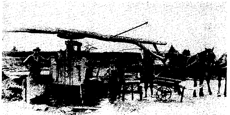
Figure 2. Pug mill, Elbridge Gage brickyard, Bellamy River, Dover, New Hampshire, c1900. This mill was turned by a team of two horses, hitched to a crude sweep fashioned from a forked tree trunk. The man at the left stands in a tempering pit; those at the right have two-wheeled handcarts for carrying off filled brick molds. Whitehouse Collection, Woodman Institute, courtesy of Thom Hindle.
