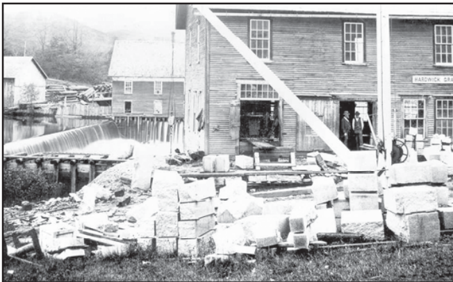
Figure 2. Riverside Granite Polishing Mill Powered by Water Turbine, Hardwick Granite Co., Hardwick, VT.
