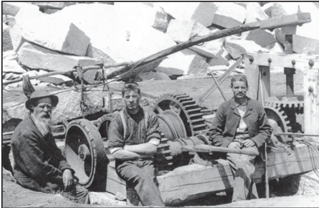
Figure 1. Horse Sweep-Powered Derrick Hoist, Barre, VT.
