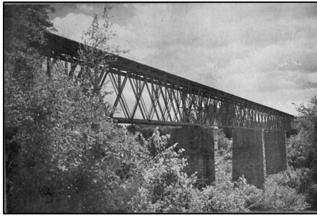
Left: The riveted iron lattice deck truss bridge that replaced the original wooden superstructure in 1889. The riveted lattice truss, the first widely popular metal railroad truss type, was widely employed on American railroads in the last decades of the nineteenth century.
