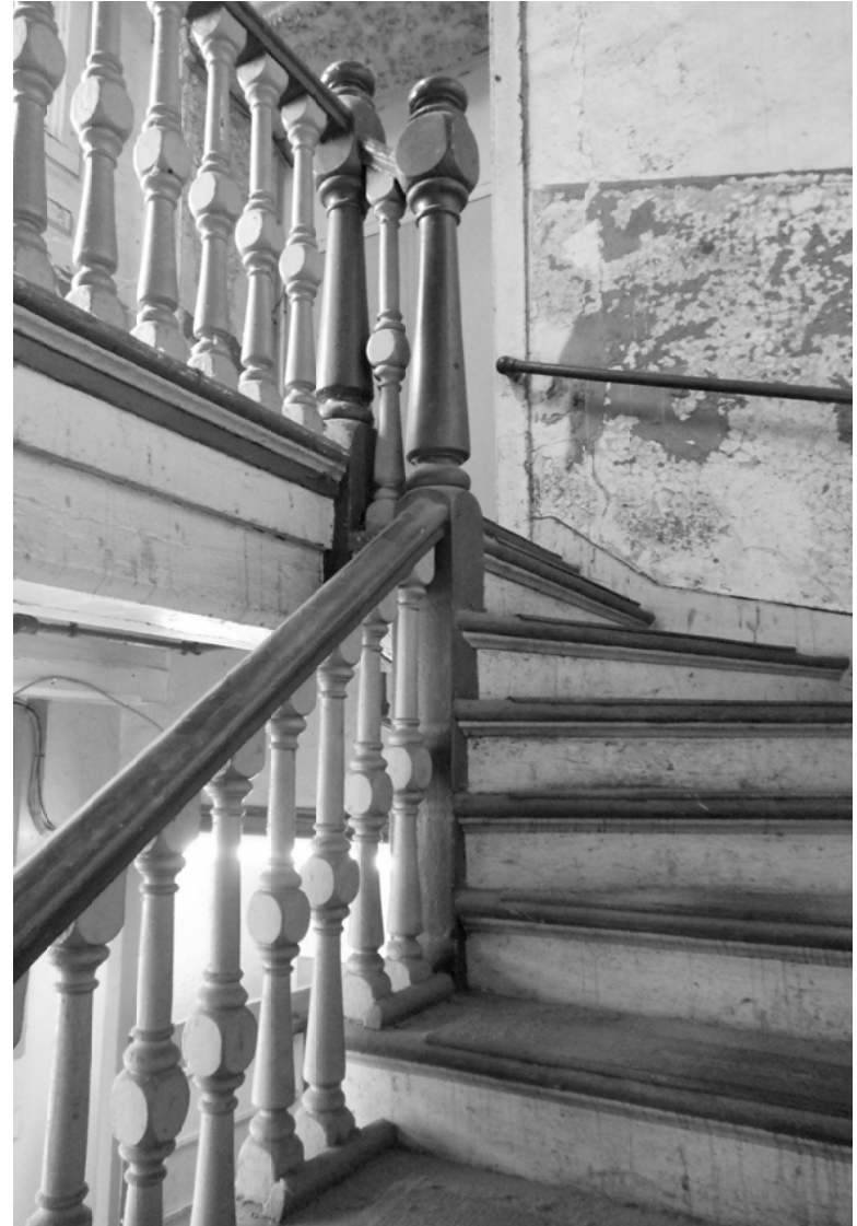
Inside the stair tower of Durfee Mill No 1 (1866)
