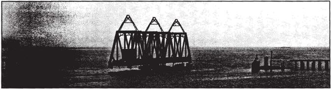
The Grand Trunk Railroad built a long timber pile bridge, with a central steel swing span, to carry its trains across the mouth of Back Cove to its station on India Street on the Portland waterfront. Part of the bridge suffered serious damage from fire in 1984, and has been out of service since then. Nelson Lawry photo.
