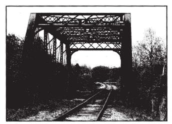
Two views of the Atlantic & St. Lawrence Railroad's steel through-truss bridge spanning the Royal River in Yarmouth, Maine. In the photo on the left, note the space on the left once occupied by a second track.. Nelson Lawry photo.
