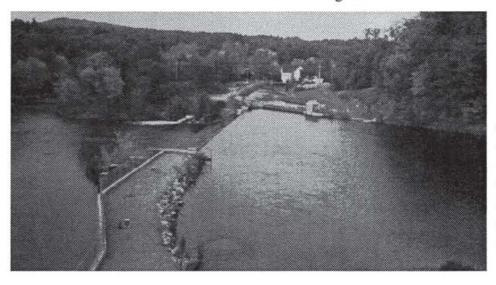
A view downstream from the top of the Hopkinton flood-control dam where a second, hydropower dam is seen. A canal supplying the hydroelectric generation station is in the distance, beyond the spillway.
