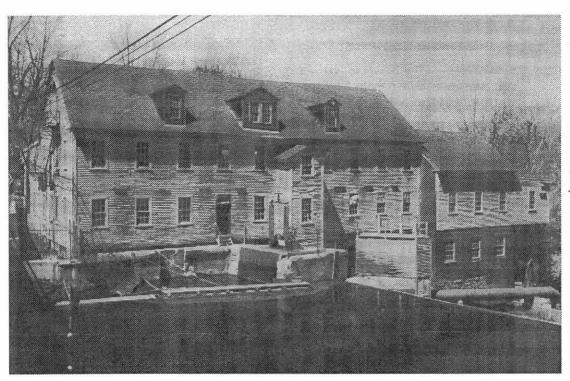
Fig. 3 The Burleigh woolen mill was constructed during the 1850s at Rocky Gorge, South Berwick, ME, using the falls of the Great Works or Asbenbedic River for the essential waterpower. The main mill building shown is a unique clapboard- overbrick construction. Th6 Great Works mill site is one of the oldest in Maine, in use since the mid-17th century.
