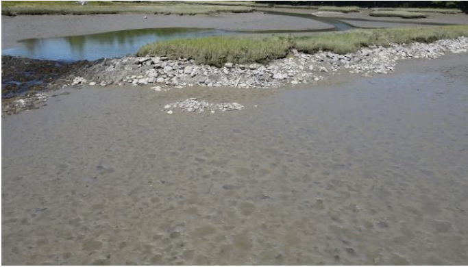
Fig. 5. Drone photo of the OMC dam showing soil cover topped with upland grass and lag deposits of stones from the eroded dam. The stones range in size from hand-size to small fragments. (Photo by Jim White, Spruce Creek TV)
