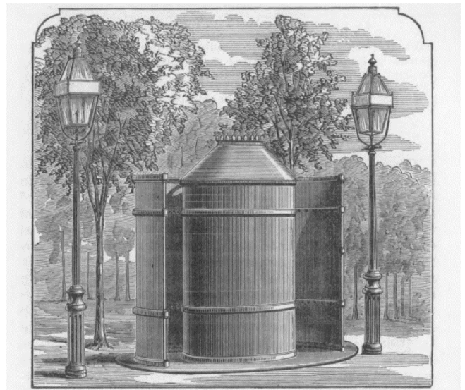
An iron "comfort station" in Boston
