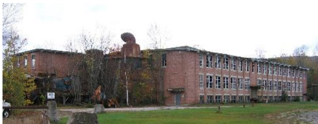
Remains of the bobbin plant
