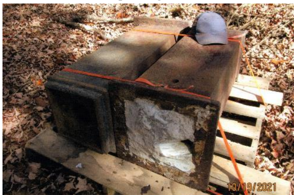
Cast-iron pillars supporting roof pillars
