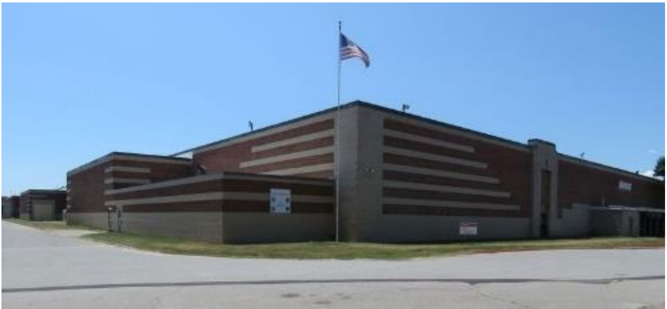
Fig. 2. Simonds Saw plant, Intervale Rd., Fitchburg showing the front (north) and east facades, in 2016. The one-story structure on the front left was added after original construction.
