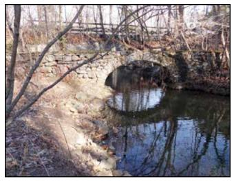
Figure 10. Downstream fascia of stone arch dike along West Brothers Brook.
