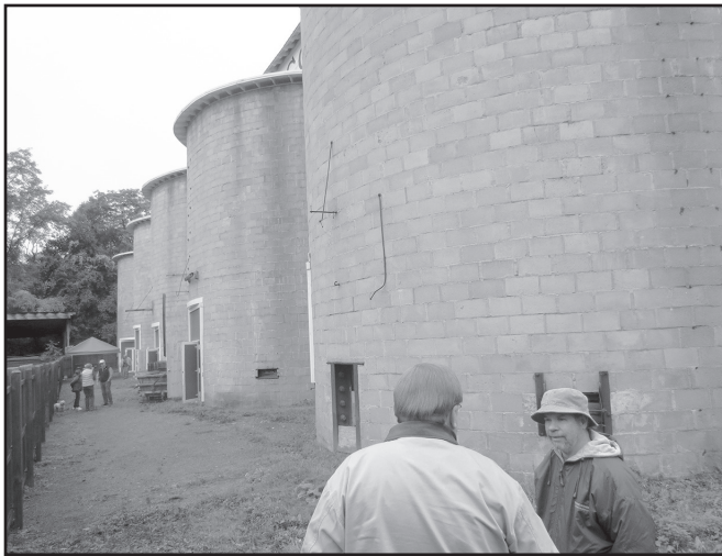
Figure 1A. Tour participants prepare to enter a renovated silo.
