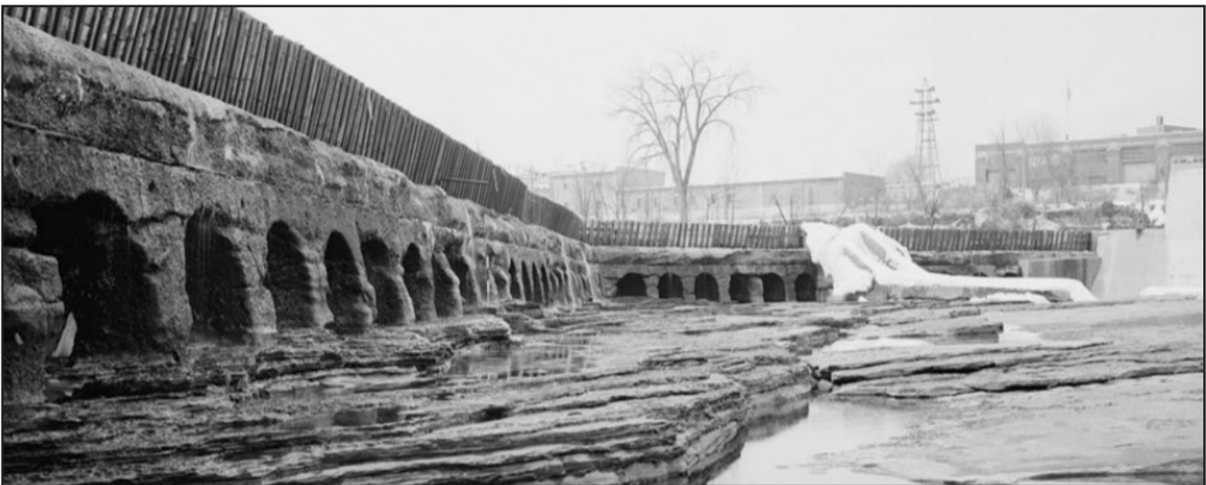
Figure 5. General view of the Glens Falls Dam from the vicinity of the southeast end, (Historic American Engineering Record, 1968, Library of Congress.)
