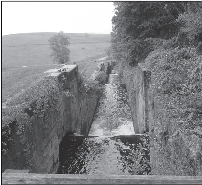
Figure 3. A down-stream view of the 7-mile long, ca. 1822 Feeder Canal that delivers water from the Hudson River to the Champlain Canal.
