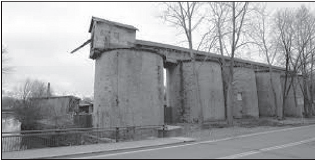
Figure 1. Concrete silos built in Glens Falls, NY, by the former Griffin Lumber Co. in 1901 to store coal. The coal was delivered by canal boat and brought to the top of the silos by conveyor to a small rail car that was run across the tops to deliver the various grades of coal to the appropriate silo. ( The Post Star photograph.)
