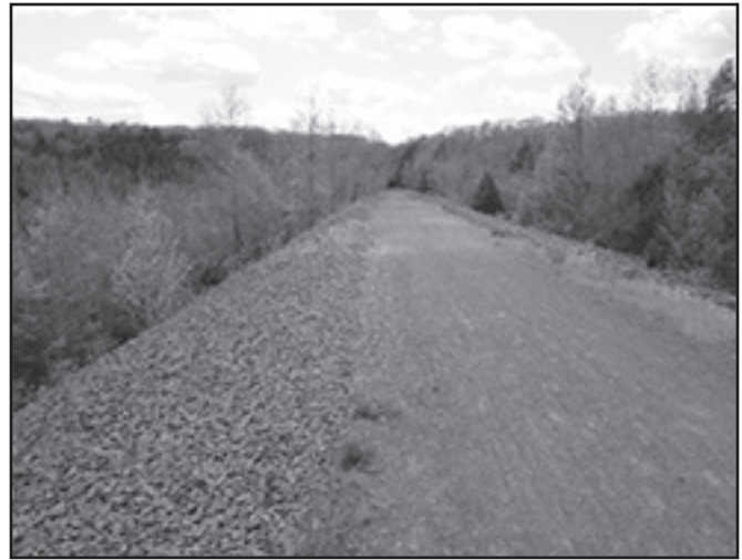
Lyman and Rapallo Viaducts, Colchester and East Hampton
