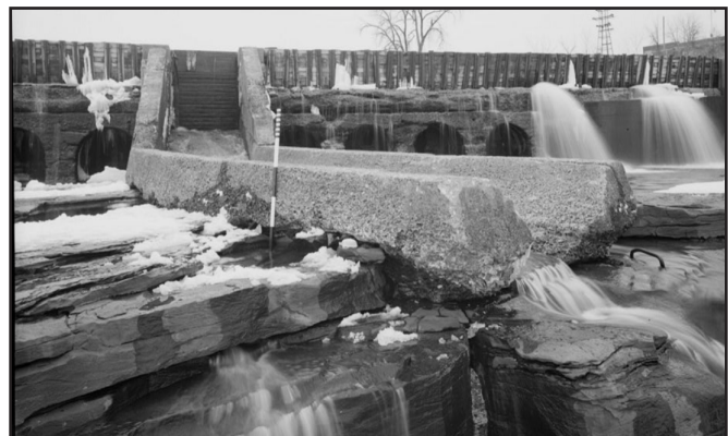
Figure 7. A closeup view of the log chute showing the turn below the Glens Falls Dam. (Historic American Engineering Record, 1968, Library of Congress.)
