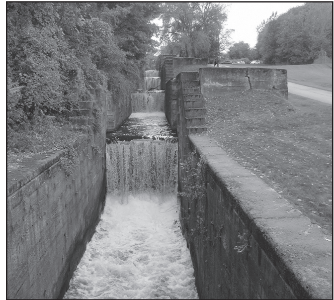
Figure 3. An up-stream view of the 7-mile long, ca. 1822 Feeder Canal that carries water from the Hudson River to the Champlain Canal.
