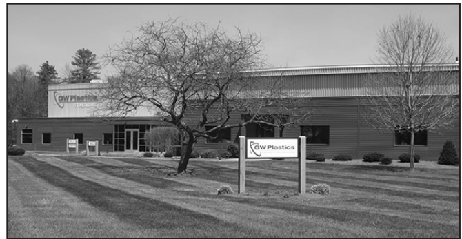
The GW Plastics plant in Bethel, Vermont.
