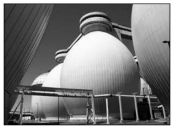
Fig. 4. Walking amongst the digesters. Each is about 90 feet in diameter and 130 feet tall made of boiler steel. Most were built by the Chicago Bridge & Iron Co.
