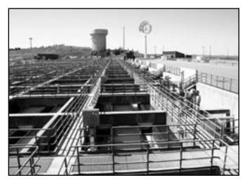
Fig. 3. Looking north over the tanks for primary clarifiers, secondary reactors, and secondary clarifiers, with a water tower and wind turbine in the distance.
