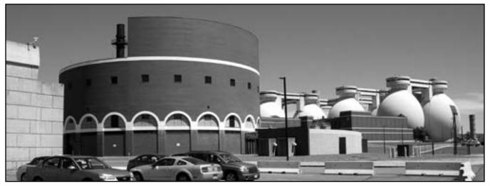
Fig. 2. The round brick building is the South System Pump Station; beyond it are odor control and centrifuge buildings and egg-shaped digesters rising in the distance.
