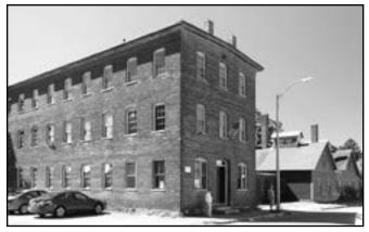
At left, the main three-story brick building of M.M. Rhodes & Sons, Inc., built in 1880. The older wooden building on the right dates from the 1850s. It was originally an umbrella factory, purchased by Marcus Morton Rhodes in the 1860s and adapted as a "Japanning house" for finishing small metal items and papier-mâché shoe buttons, which was the company's primary product for many years.
