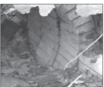
Detail of the fire brick lining of the Taylor electric furnace. A 2012 photo.
